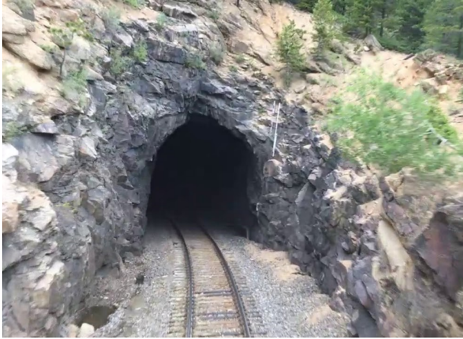
A Typical Tunnel
