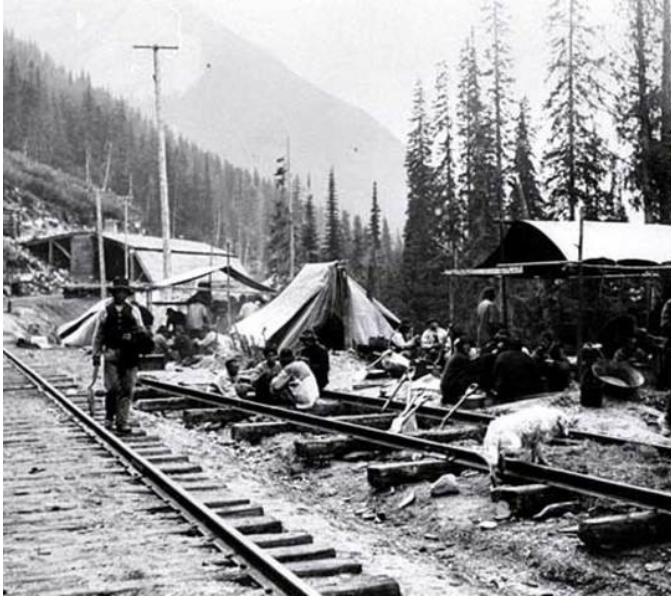
A Railroad Work Crew
