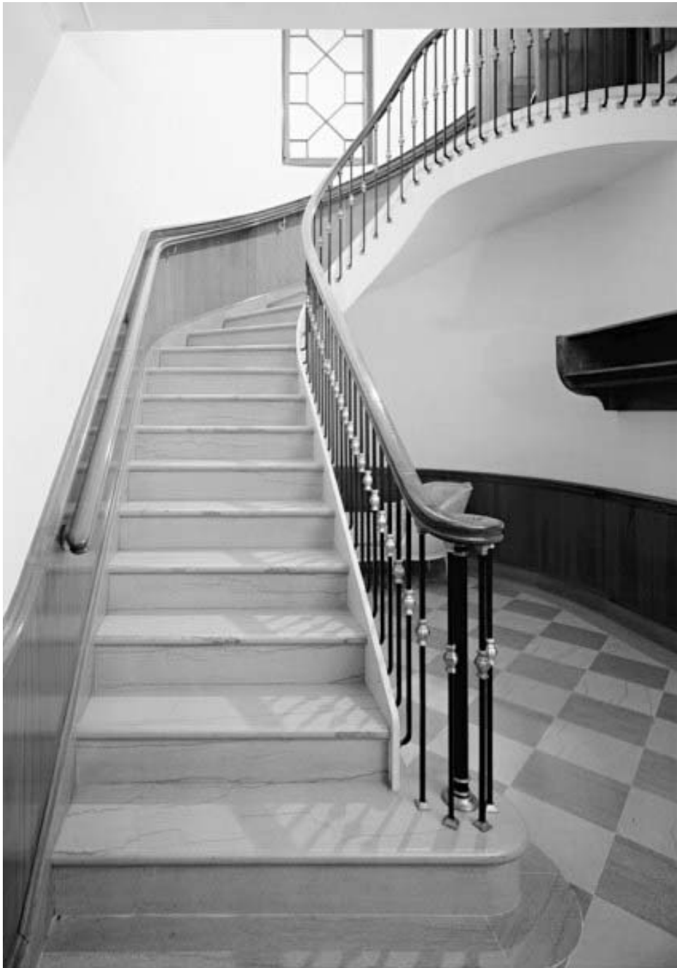
Figure 4: Stair to the Containment Area
